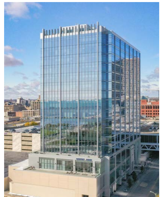
PBDC's new office space at 833 East Michigan
