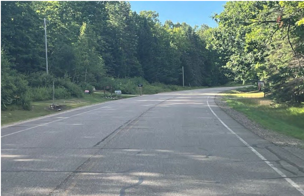
Horizontal curve on County W without enhanced signing and marking
