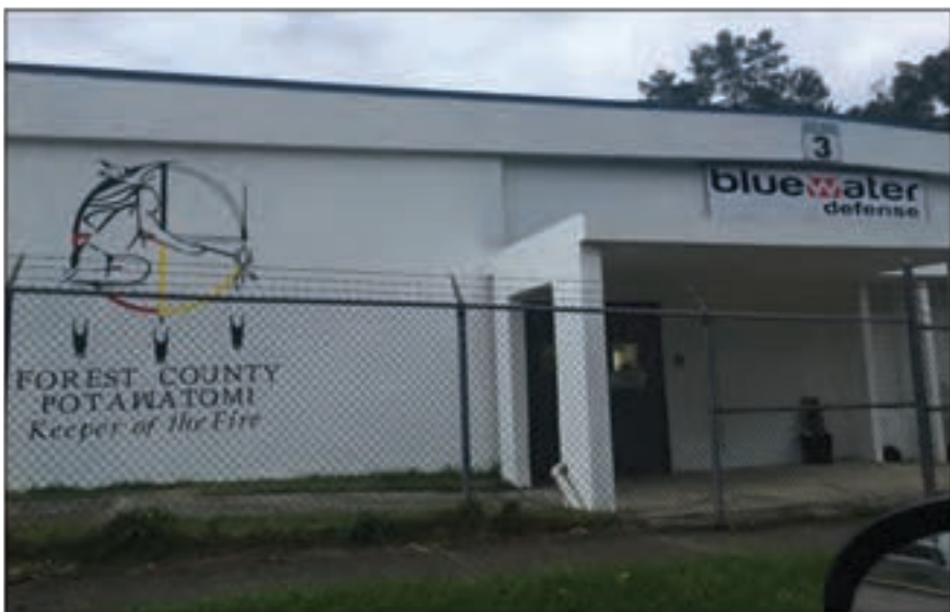
Pictured above: Exterior photo of the manufacturing building branded with FCP logo.
