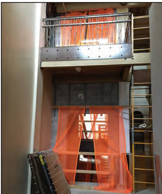
Elevator installation in the main lobby area.
