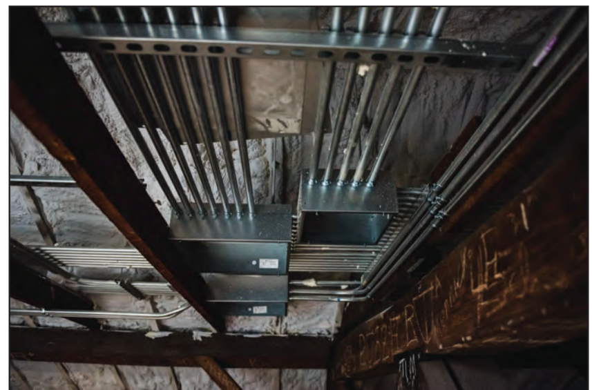
Electrical conduit installed on the third floor attic space.
