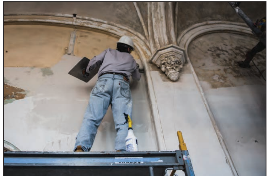
Plaster repairs on the second floor.
